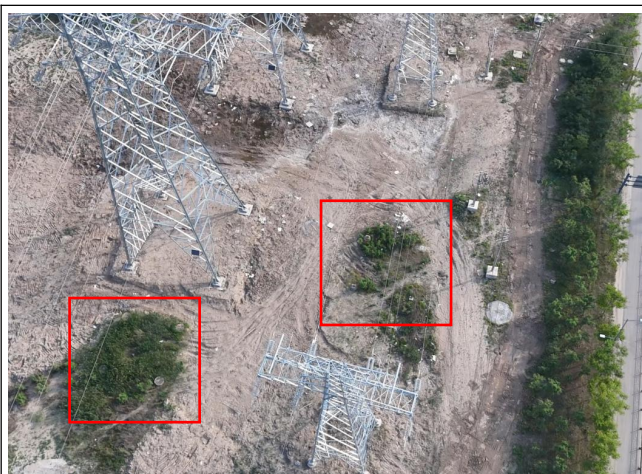
拆除杆塔周围生态恢复
